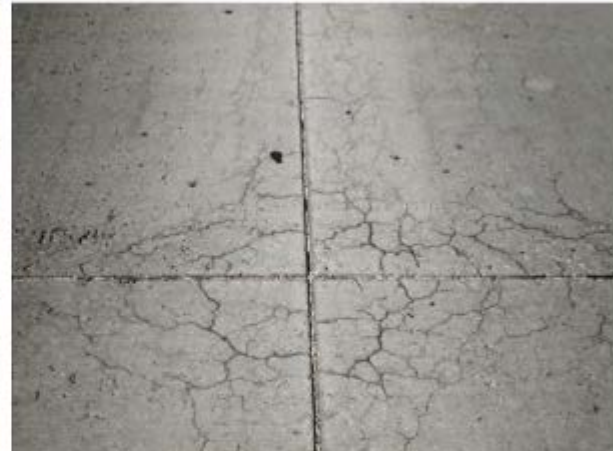
Alkali Silica Reactivity ( www.fhwa.dot.gov )
