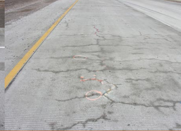
Shrinkage Cracking ( www.carasquilloassociates.com )
