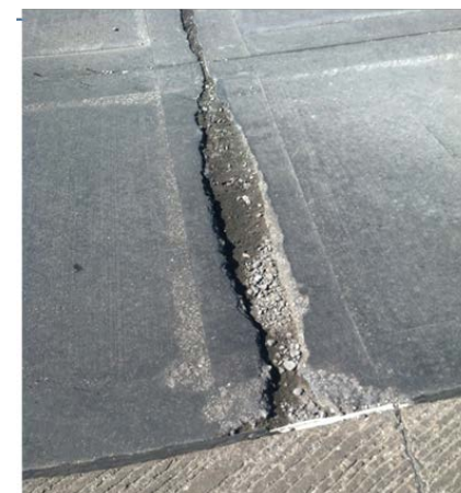
Joint Damage (Weiss et al. 2005, Byers 2015)
