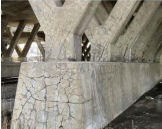
Alkali Silica Reactivity ( www.fhwa.dot.gov )
