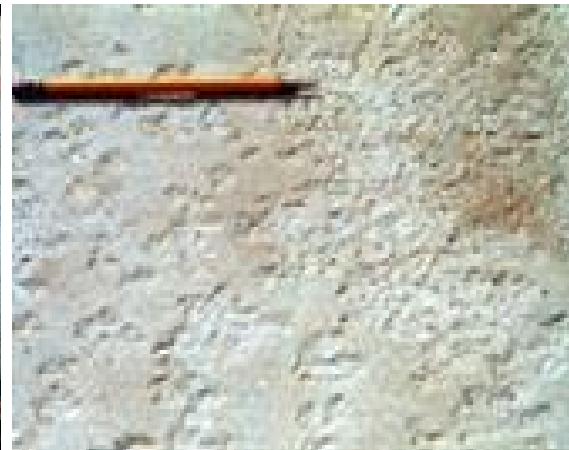
Freeze-Thaw Damage ( www.cement.org )
