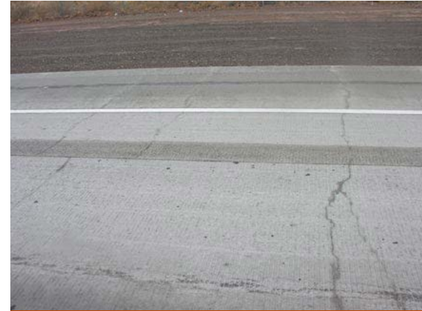
Shrinkage Cracking ( www.carasquilloassociates.com )
