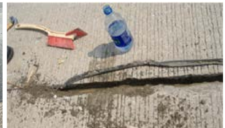
Joint Damage (Weiss et al. 2005, Byers 2015)
