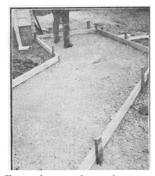
There are three areas of concern for non-uniformity of sub-bases that will cause the slab to discolor due to different water/cement ratios. One, it is critical the sub-base be uniform in its composition. For example: when 3/4" minus aggregate is used, there should not be areas that are finer than others. Two, the thickness of the sub-base must be uniform, and three, that it is leveled so the concrete will be the same thickness.
